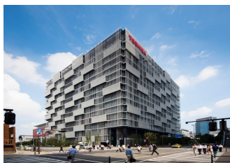
Leased new facility provides highly functional new corporate offices
