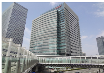
Purchased new facility provides highly functional new corporate offices
